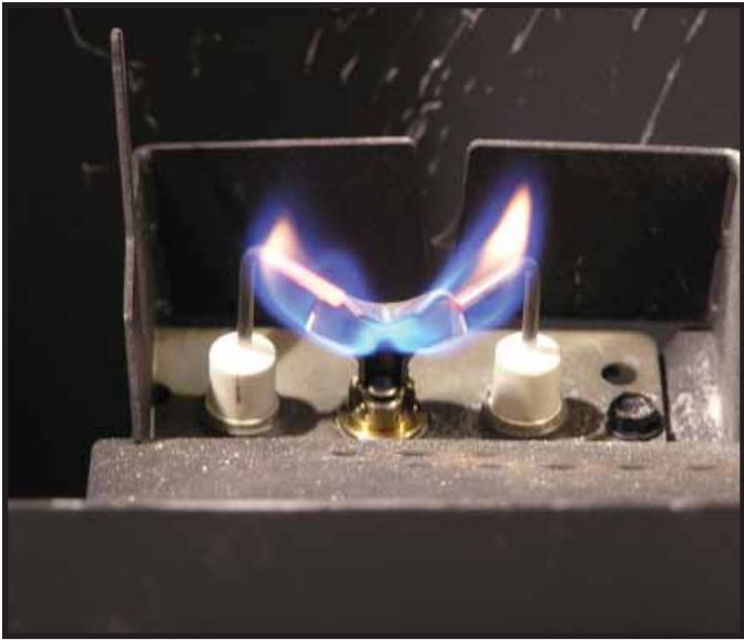
Figure 3.1 IPI Pilot Flame Patterns
