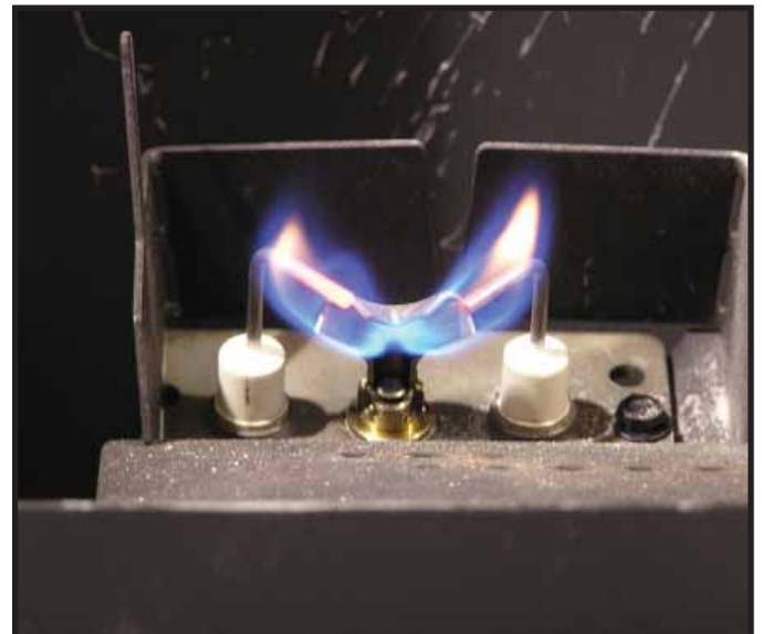
Figure 4.5 IPI Pilot Flame Patterns
