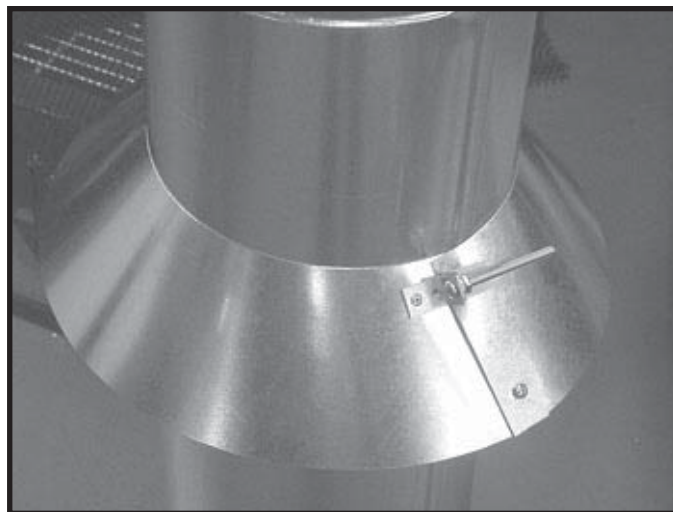
Figure 8.19 Assembling the Storm Collar Around the Pipe
