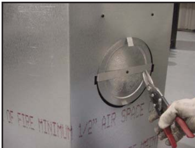
Figure 7.7 Cut the metal retaining band and fold the sides out.
