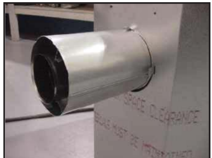
Figure 7.10 Attach the first vent section (it will snap into place). Slide the insulation gasket onto the vent section, up against the appliance and over the tabs.
