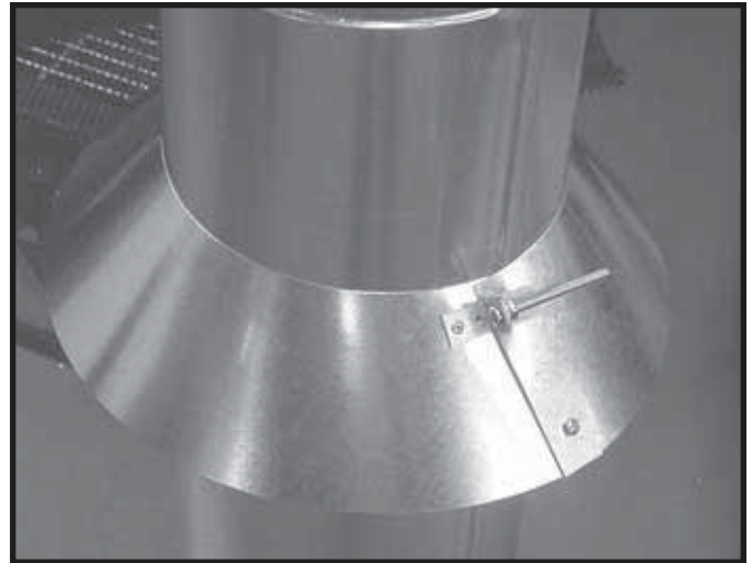
Figure 8.18 Assembling the Storm Collar Around the Pipe
