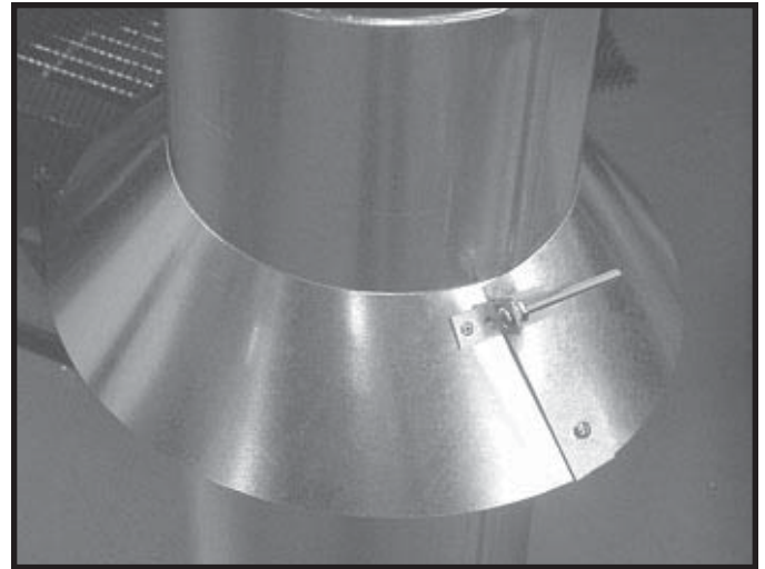
Figure 8.8 Assembling the Storm Collar Around the Pipe
