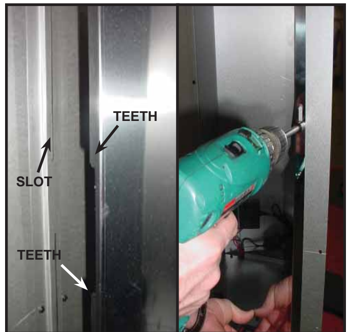
Figure 14.6 When screwing the panel in place start with the center screw and with your free hand lift the panel up so that it comes in contact with the top reflector panel. Insert all screws until finished.
