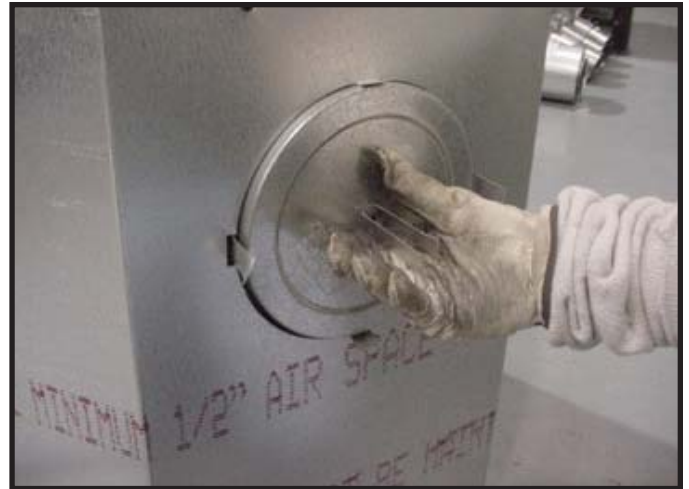
Figure 7.8 Fold the center parts of the retaining band out and use to remove the vent cap.
