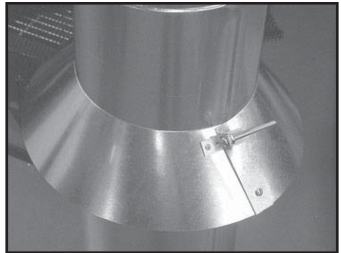
Figure 8.20 Assembling the Storm Collar Around the Pipe
