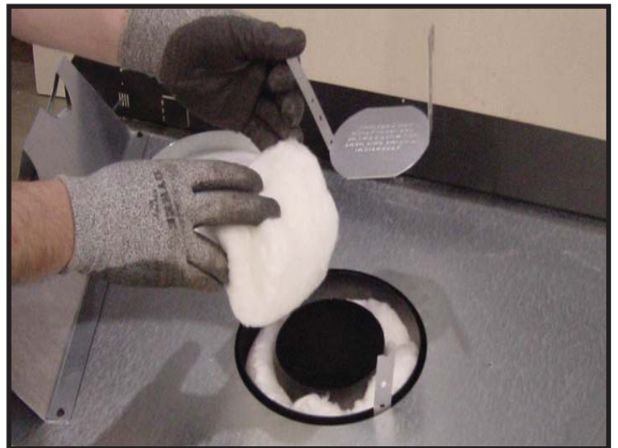
Figure 7.5 Remove the insulation basket and white insulation from the center vent pipe.
