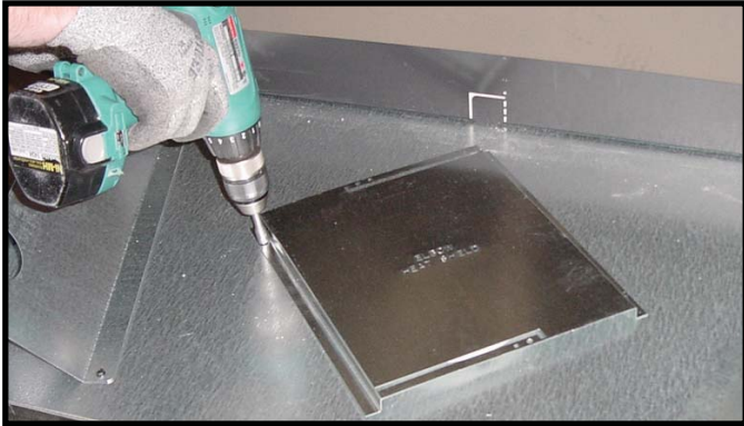
Figure 7.1 For top vent, remove the two screws holding the elbow heat shield in place. Use this heat shield over the first elbow if applicable. For rear vent skip this step.
