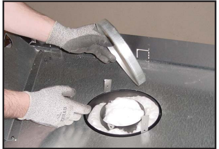
Figure 7.4 Remove the seal cap.
