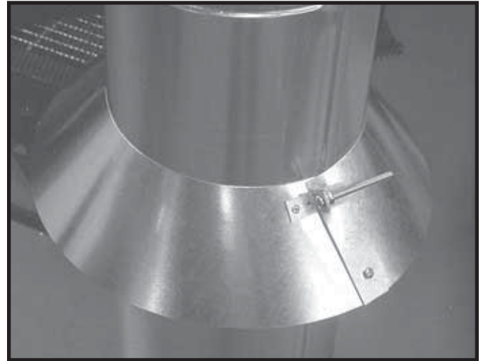
Figure 8.18 Assembling the Storm Collar Around the Pipe
