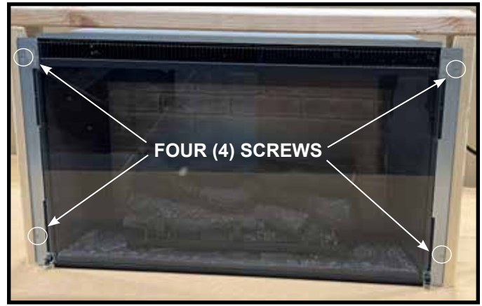
Figure 4.9 Fastening Framing Tab to Framing
