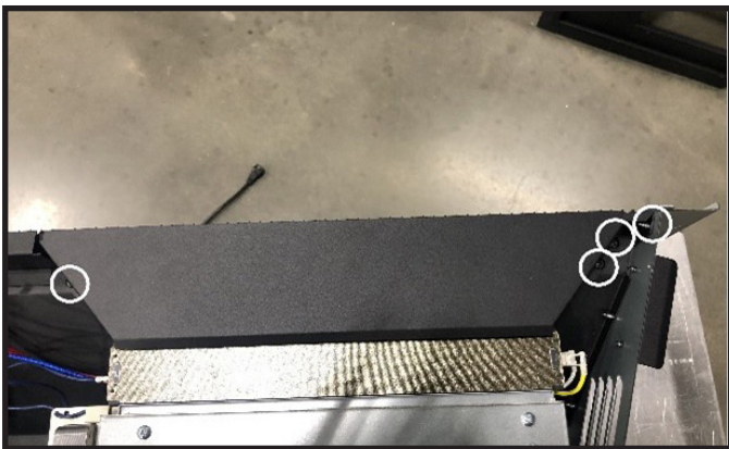
Figure 6 Heater Shroud Removal
