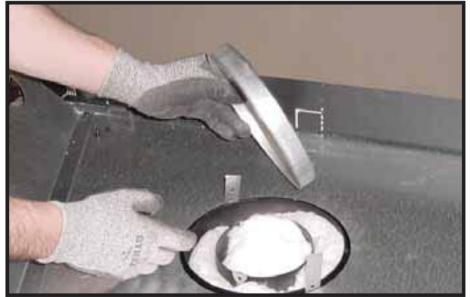
Figure 7.4 Remove the seal cap.
