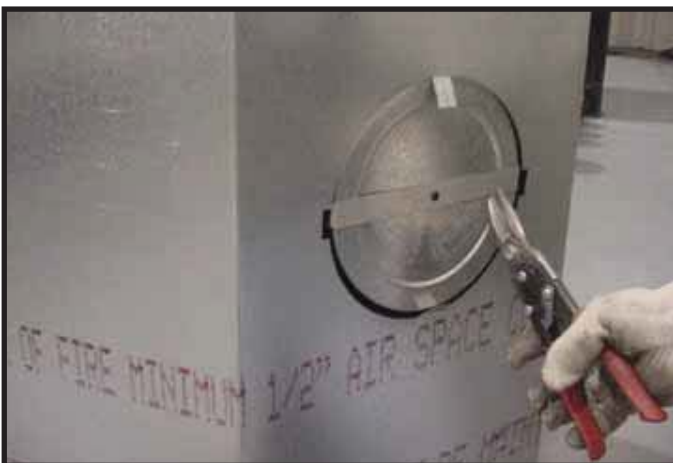
Figure 7.7 Cut the metal retaining band and fold the sides out.
