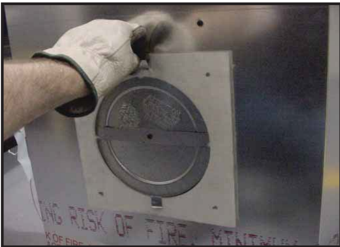
Figure 7.8 Fold the tabs toward the center of the fire plug (90°) and remove the insulation gasket.
