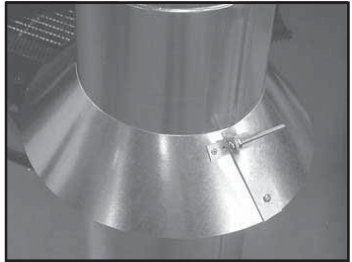
Figure 8.20 Assembling the Storm Collar Around the Pipe
