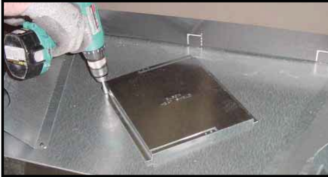
Figure 7.1 For top vent, remove the two screws holding the elbow heat shield in place. Use this heat shield over the first elbow if applicable. For rear vent skip this step.
