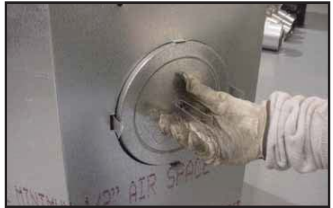
Figure 7.10 Fold the center parts of the retaining band out and use to remove the vent cap.
