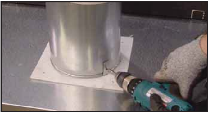
Figure 7.7 To attach the first section of vent pipe, make sure to use the fiberglass gasket in the manual bag to seal between the first vent component and the outer fireplace wrap. Use 2 self tapping screws to secure the gasket to the outer wrap.
