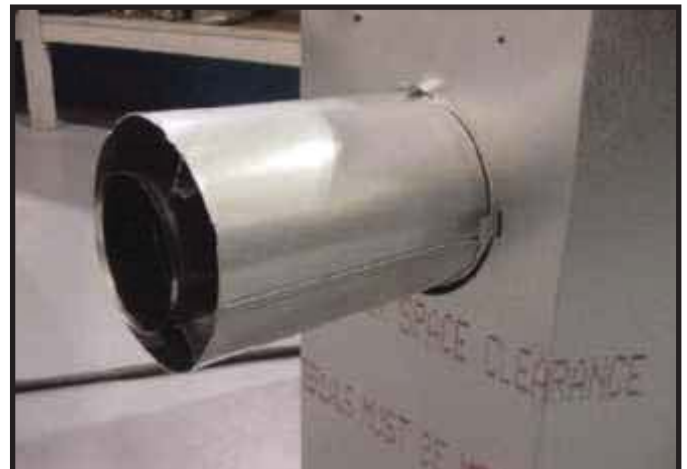
Figure 7.10 Attach the first vent section (it will snap into place). Slide the insulation gasket onto the vent section, up against the appliance and over the tabs.
