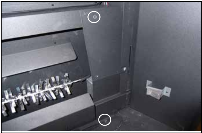
Figure 16 Removal and installation of faux flame access panel.
