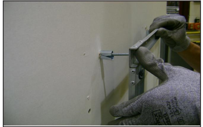
Figure 4.6 Installing Anchors in Hollow Wall
