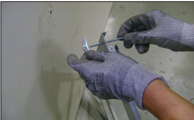
Figure 4.5 Toggle Bolt Installation through Mounting Bracket
