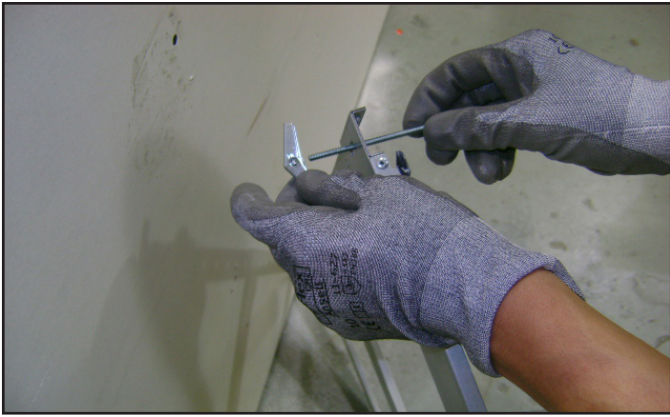
Figure 30 Toggle Bolt Installation through Mounting Bracket
