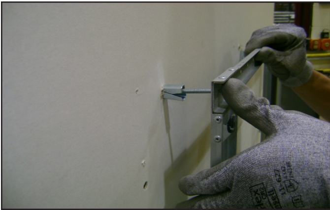
Figure 31 Installing Anchors in Hollow Wall
