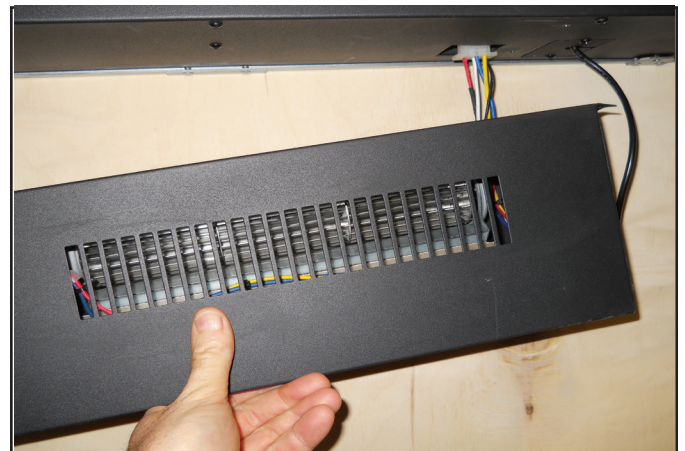
Figure 15 Support Fan Box while accessing Electrical Connector
