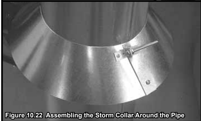
Figure 10.21 Assembling the Storm Collar
