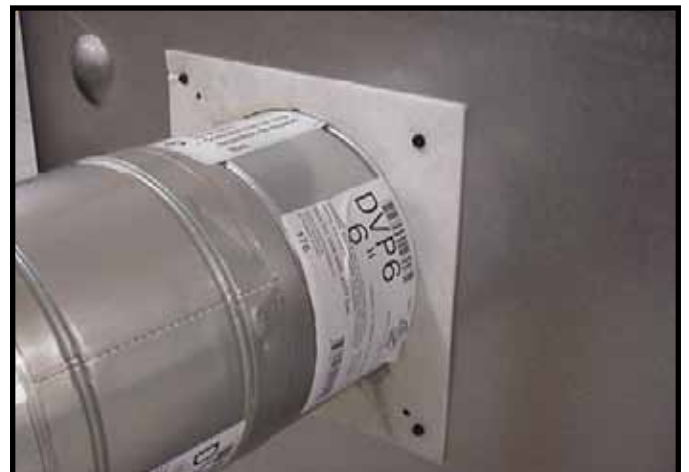
Figure 9.12 Attach the first vent section (it will snap into place). Slide the insulation gasket onto the vent section, up against the appliance and over the tabs. Use two self-tapping screws to secure gasket to outer wrap.
