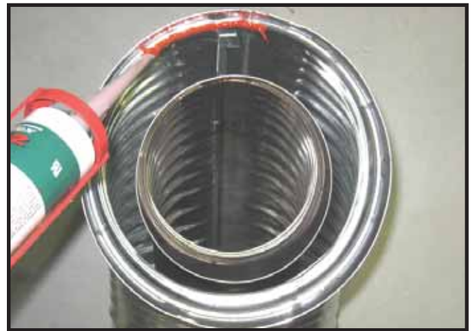
Figure 8.2 High Temperature Silicone Sealant
