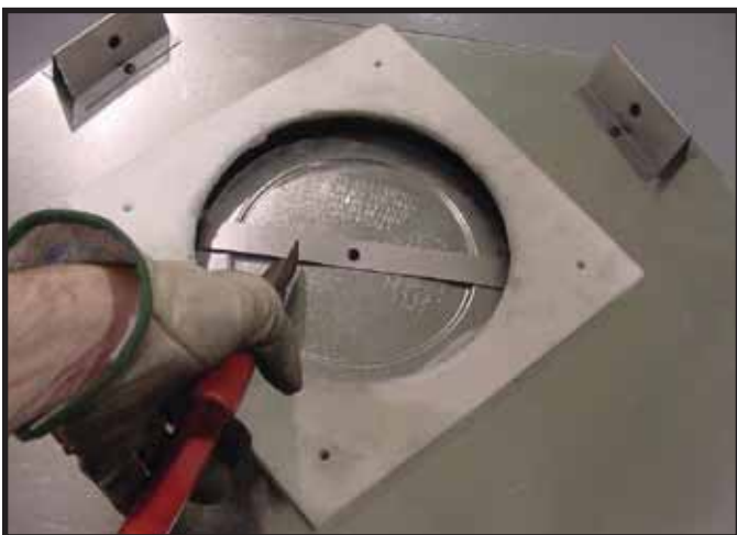
Figure 7.3 Cut the metal retaining band and fold the sides out.
