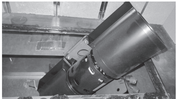
Figure 4.14 Remove Fan from Access Hole
