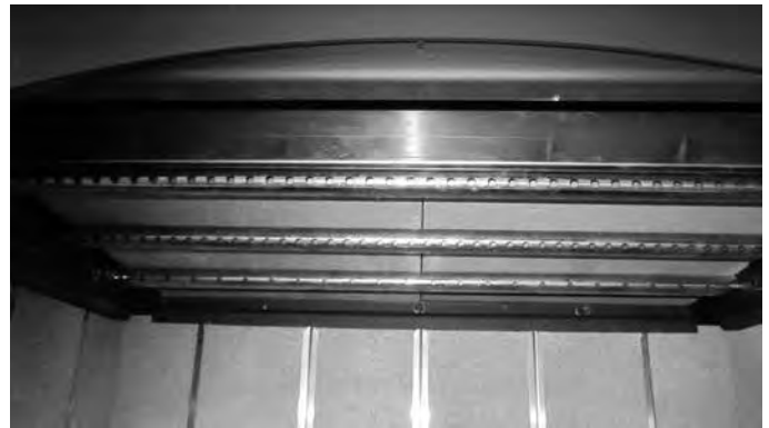
Figure 4.8 Reinstall Baffle Boards
