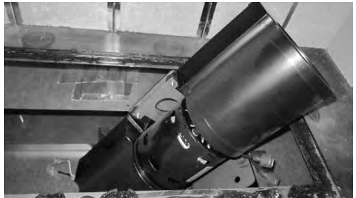
Figure 4.14 Remove Fan from Access Hole
