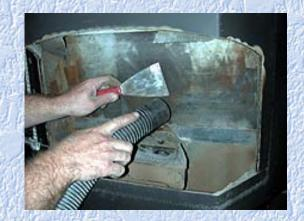
Scrape any carbon deposits from the burn pot. You will find that a standard screwdriver and hammer works best for this.
