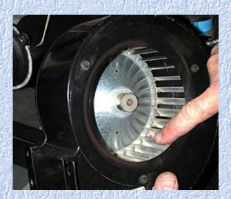
Remove the screws holding the blower in place using a socket wrench with an 8" extension. Use a toothbrush to remove dust from the fins, but be careful not to bend any of the fins. Once the fan blade has been cleaned reattach the fan.
