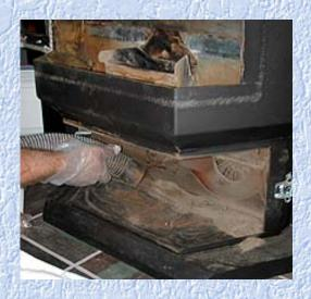
Remove the combustion blower cover plate and vacuum the fins of the combustion blower. An old toothbrush works well for removing deposits on the blower fins.
