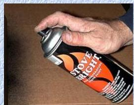
Simply shake up the can and apply a thin coat over the parts of the stove that need to be touched up. Use newspaper to mask areas and to prevent over spray. Hold the paint can upright and about 6 inches from the stove when you are painting.
