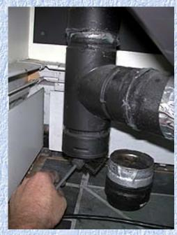
Note: Professional installers often design the venting system so that certain joints can be taken apart. These joints will often have either aluminum tape or silicone caulking on the outside. Use a knife to scrape off the silicone caulking on the joints you plan to take apart.
