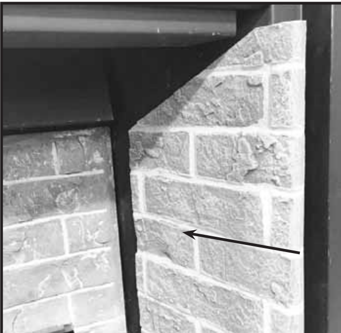
Figure 4. Install Refractory Panel (Right Side Shown)
