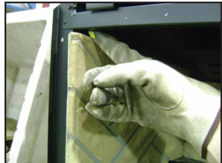
Figure 5. Bend Refractory Tab
