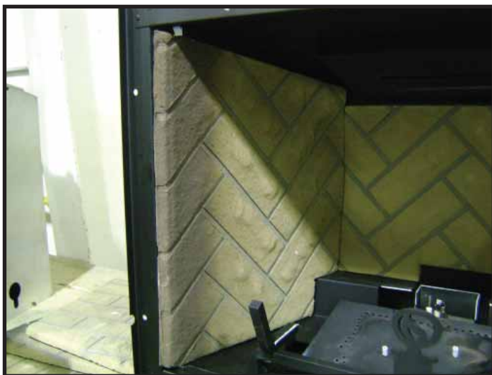
Figure 3. Install Side Refractory
