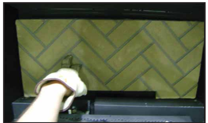
Figure 2. Install Back Refractory
