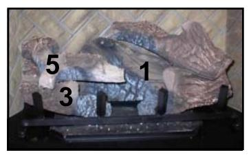
**STEP 6:** LOG #5 (SRV700-706): Place log #5 across logs #1 and #3 with the Y-shape facing out.
