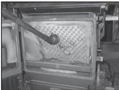
Figure 28.1 - Example of a dirty heat exchanger
