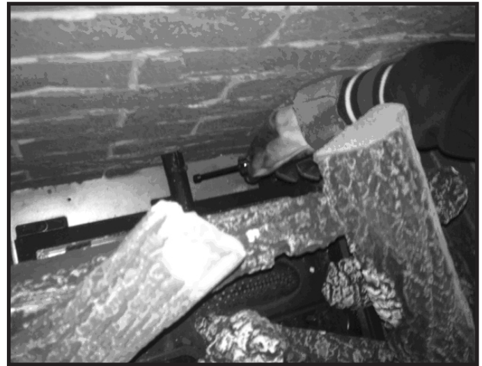
Figure 9.1. Air Shutter Location
