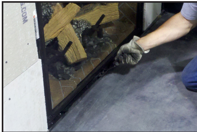
Figure 11.8. Securing Bottom Glass Clips
