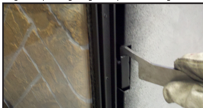
Figure 11.7. Securing Side Glass Clips
