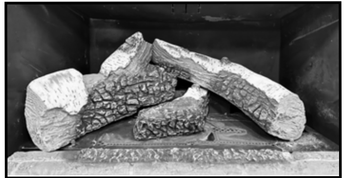
Figure 14.B Log #3 Installed (Birch Logs)
