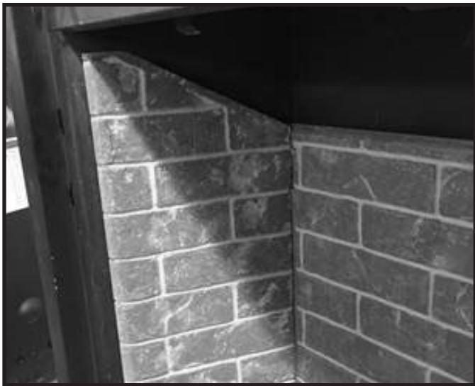
Figure 11.4 Install Left Refractory Panel
