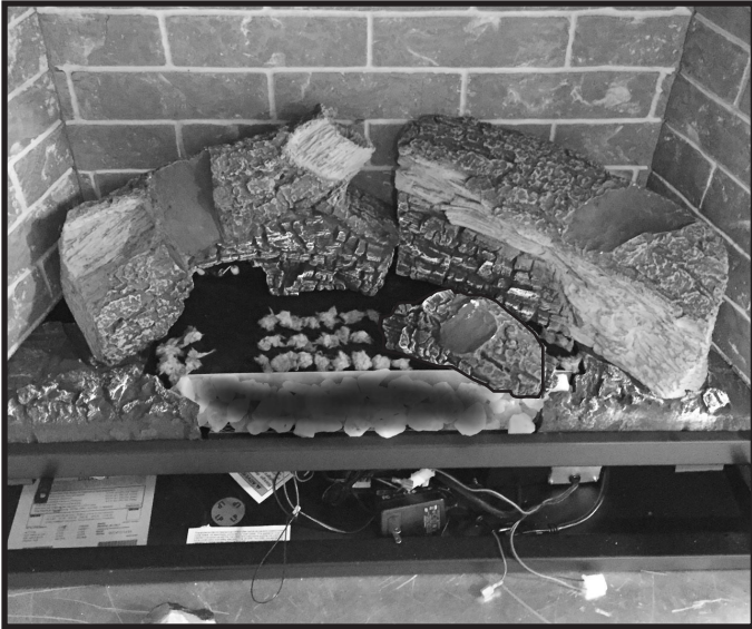
Figure 6. Burner Log Installed
