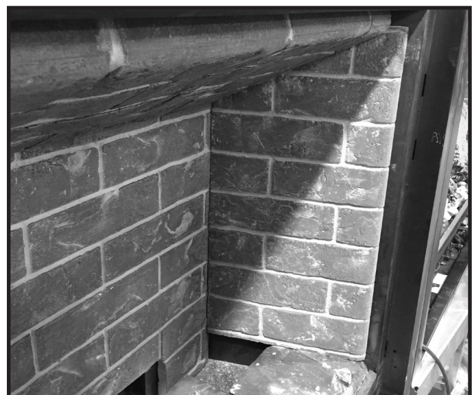
Figure 11.7 Right Refractory Panel Installed
