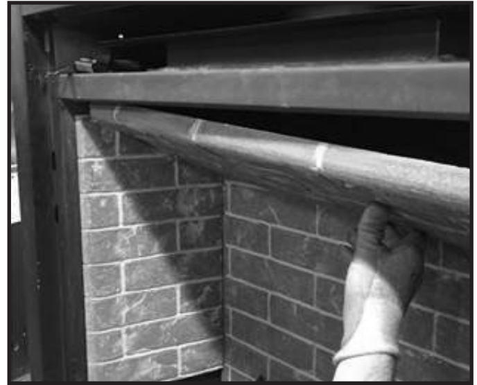
Figure 11.5 Install Top Refractory Panel
