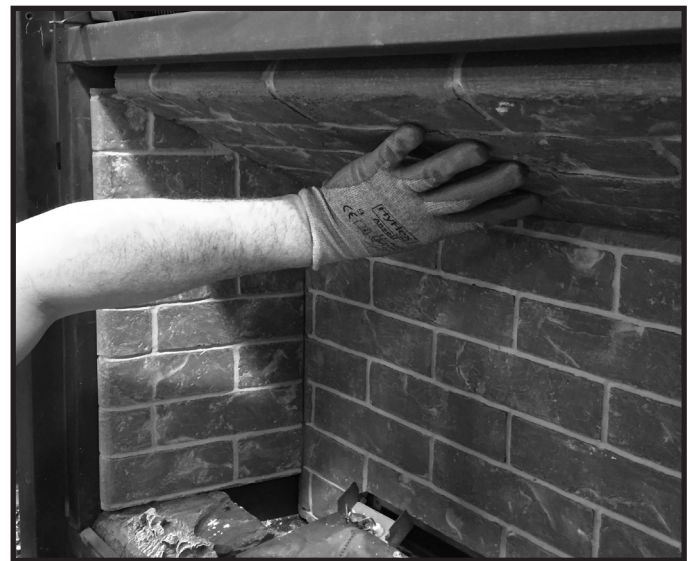
Figure 11.6 Install Right Refractory Panel
