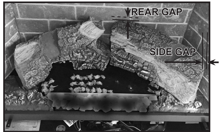
Figure 5. Rear Right Log Installed
