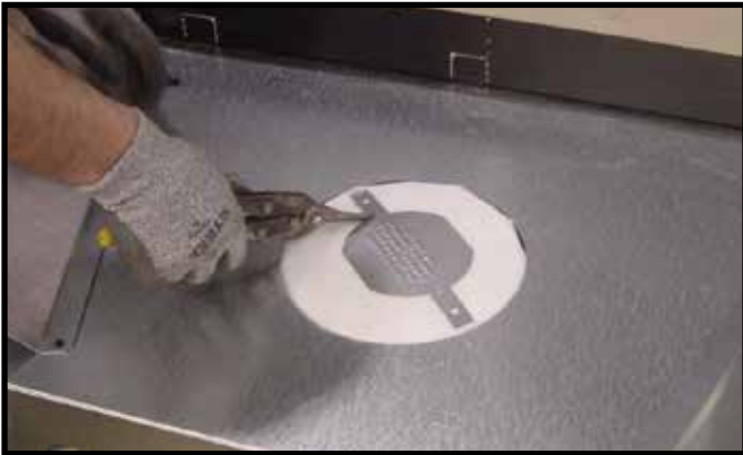
Figure 6.1 (Generic Fireplace Shown) Cut the seal cap strap across the rectangles next to the disk. For rear vent, skip this step.
