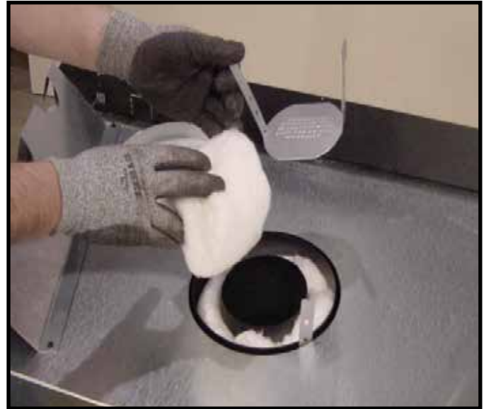
Figure 6.4 (Generic Fireplace Shown) Remove the insulation basket and white insulation from the center vent pipe.
