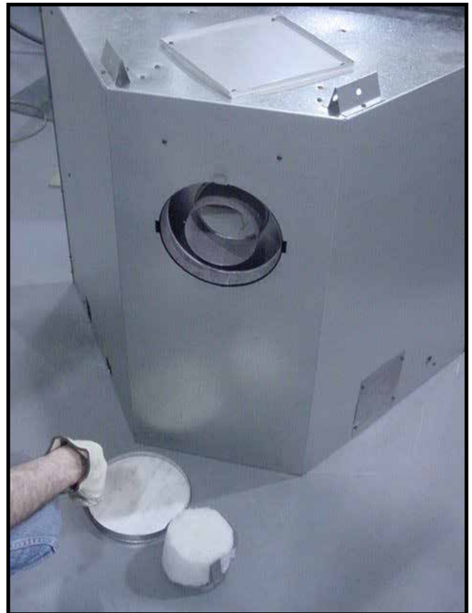
Figure 6.9 (Generic Fireplace Shown) Discard the vent cap, remove and discard the insulation basket.
