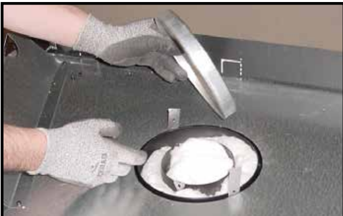
Figure 6.3 (Generic Fireplace Shown) Remove the seal cap.
