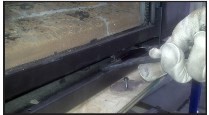
Figure 11.2. Glass Clip Tool Location
