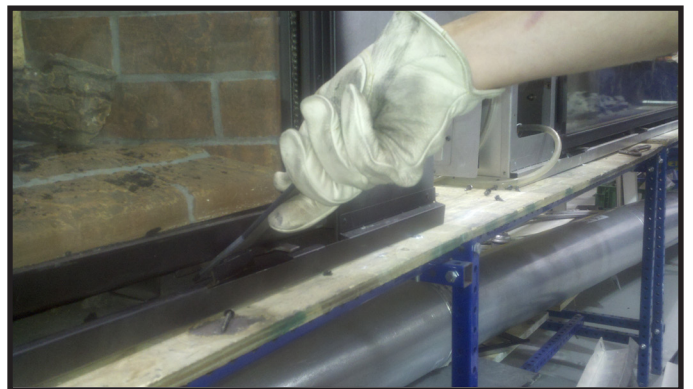
Figure 11.3. Inserting Glass Clip Tool
