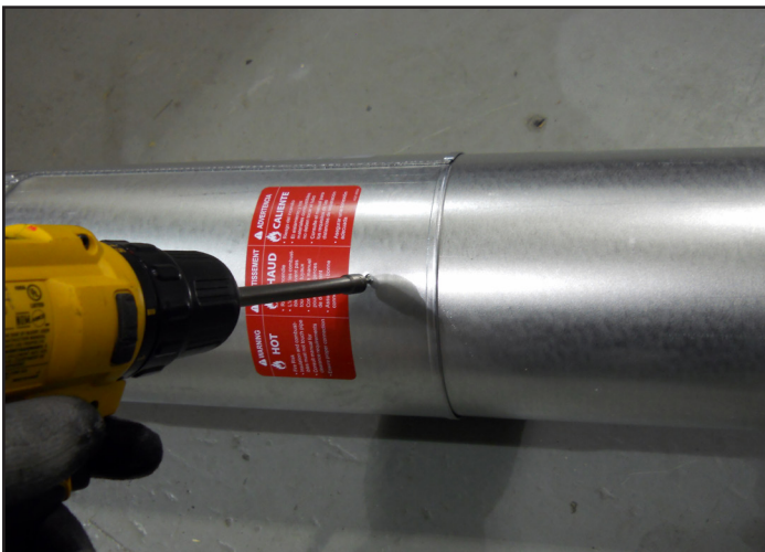
Figure 7.4 Vis de la section coulissante
