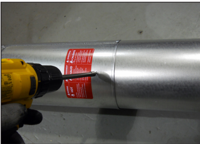
Figure 7.4 Vis de la section coulissante
