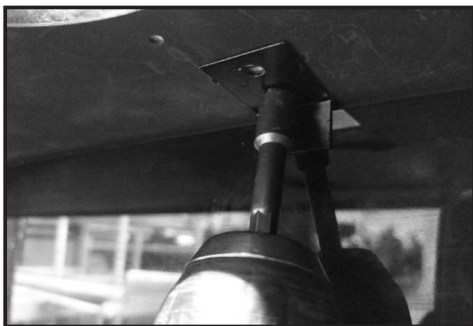
Figure 3 Installation du support de retenue - Arrière
