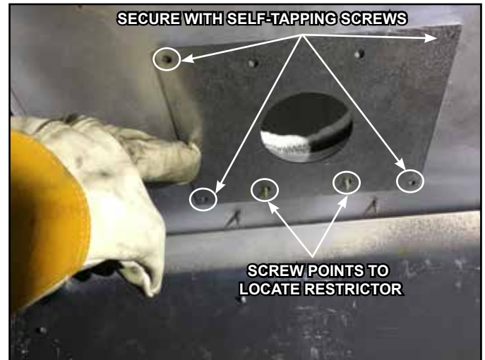
Figure 5.9 Natural Gas Restrictor Plate
