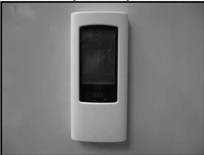
Figure 3.10 Mounted Remote Control Housing
