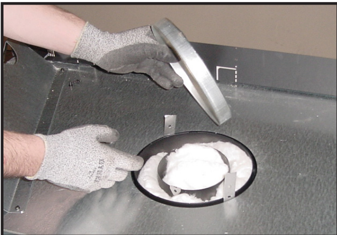
Figure 6.3 (Generic Appliance Shown) Remove the seal cap.
