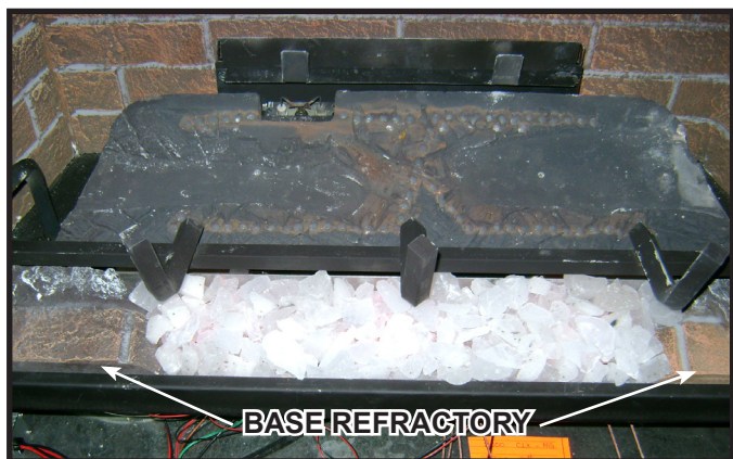
Figure 11.6 Install Base Refractory
