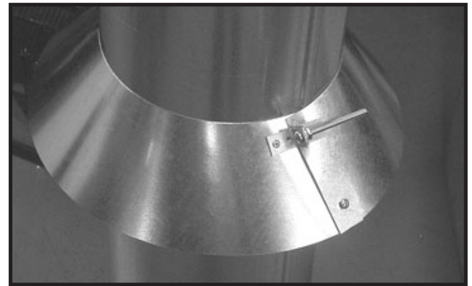
Figure 7.11 insert Bolt into Brackets
