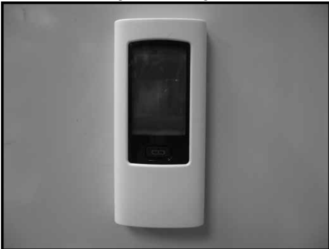
Figure 3.10 Mounting Remote Control Housing
