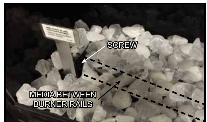
Figure 11.11 Media Placement Jig in Place
