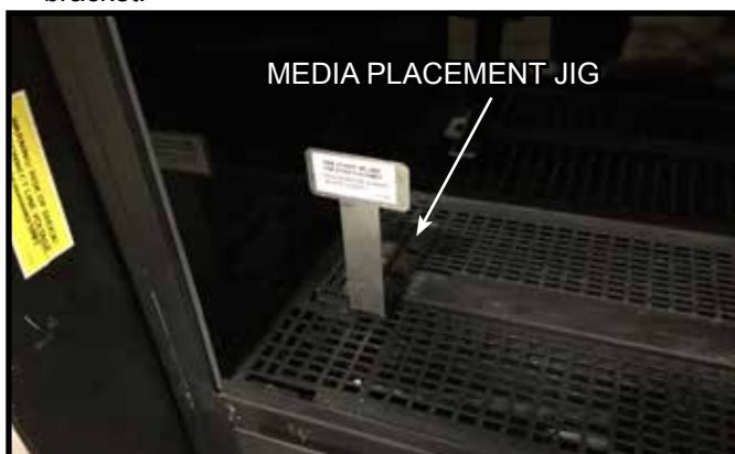
Figure 11.10 Media Placement Jig in Place
