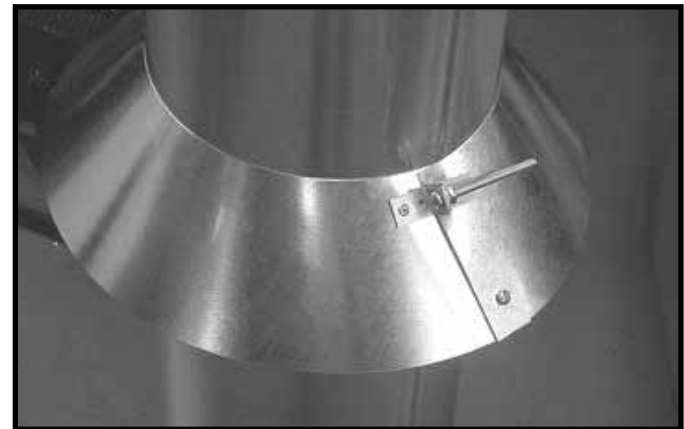
Figure 7.14 insert Bolt into Brackets
