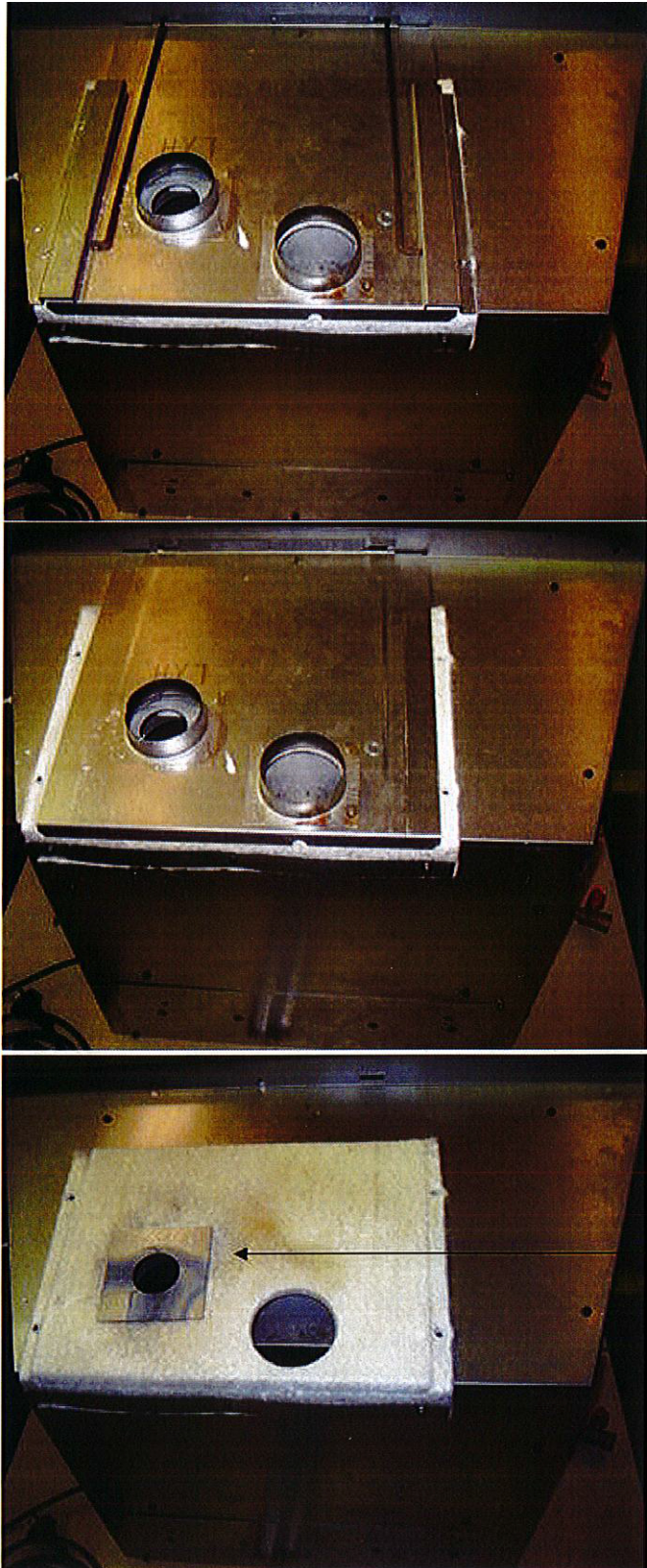
Flue baffle restrictor plate fitted to flue outlet
