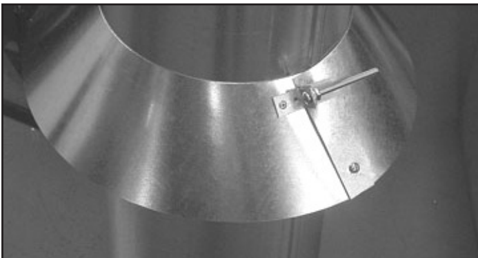
Figure 10.21 - Assembling the Storm Collar Around the Pipe
