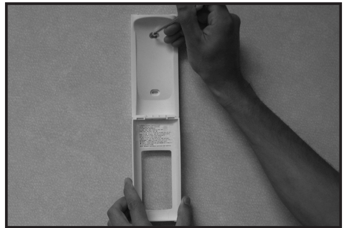
Figure 12.4 Mounting Remote Control Housing
