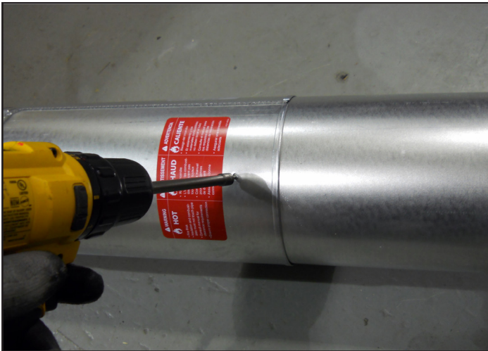
Figure 7.4 - Screws into Slip Section
