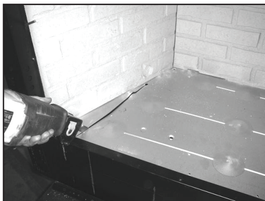
Figure 10.3. Using a saws-all, cut out the floor.
