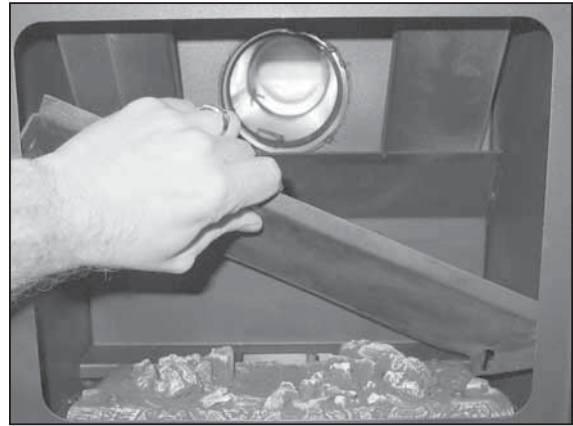
Figure 8.4 Installation of the flue restrictor requires the removal of the baffle located inside the firebox. Remove the baffle by first removing the two screws holding the baffle in place (one on each side).
