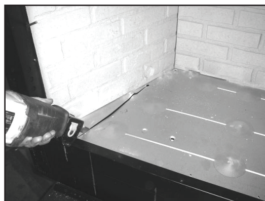
Figure 10.3. Using a saws-all, cut out the floor.
