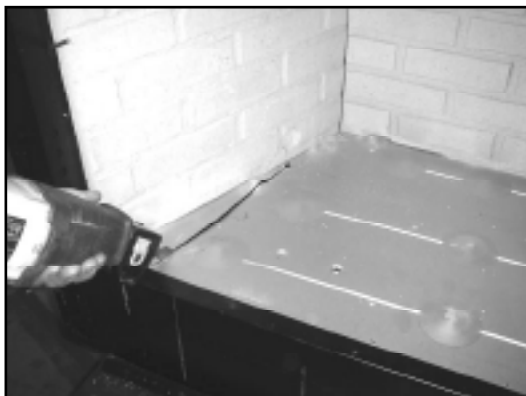
Figure 11.2. Using a saws-all, cut out the floor.
