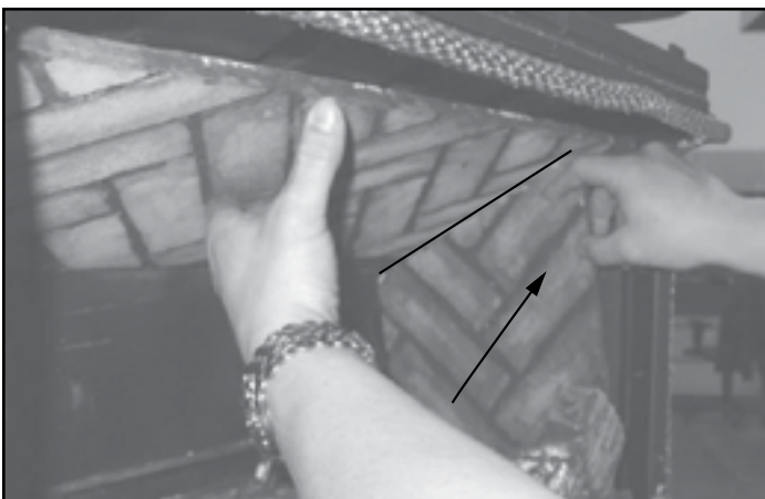
Figure 8.13 - Keeping the baffle elevated with your hand, put the right side brick into position. Rest the baffle on the right side brick.
