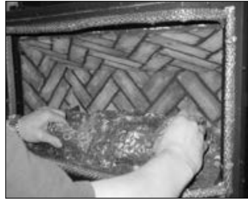
Figure 6.2 - Lift burner up and out of the firebox opening.
