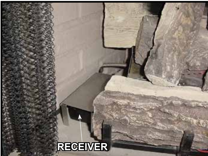
Figure 5. Receiver Location-Left Side of Log Set
