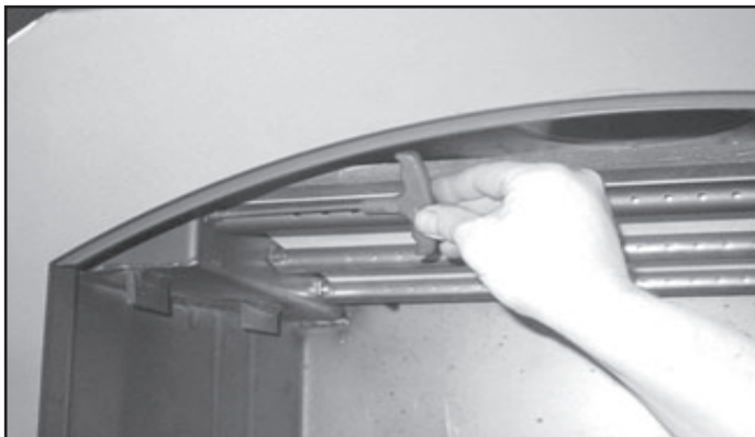
Figure 4.6 Removing Manifold Tube
